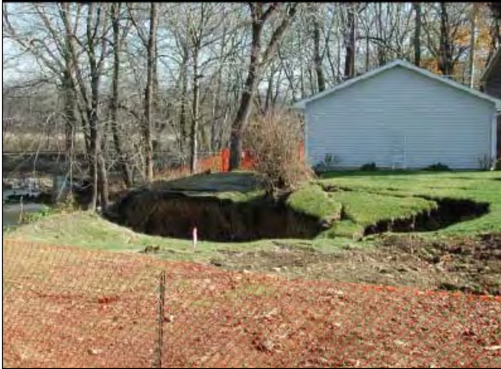
Figure 4.3.9-5. Collapse of Creek Bank and Yard along Bushkill Creek
